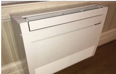
A low-wall or "floor mounted" unit can be a great replacement for an old radiator
