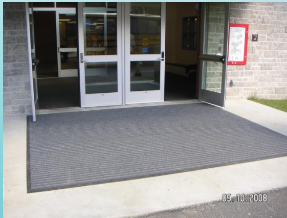
Walk off system at New Hampshire school
