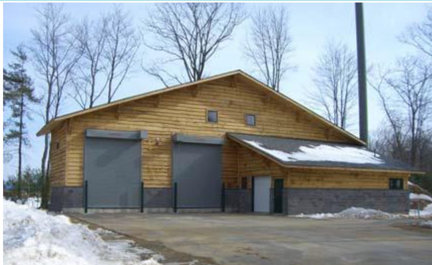
Figure: Exterior view of Merrimack Valley Regional High School (Pennacook, NH) Wood Chip Heating Plant. The smaller building near the entrance of the plant serves as the observation learning space for students and visitors.
