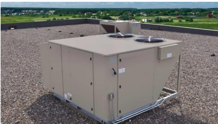
Figure 1: Typical Advanced Rooftop Unit. 12
