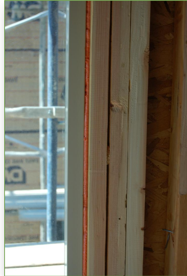
Photo courtesy of Ken Baker, K energy
