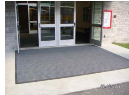
Walk off system at New Hampshire school
