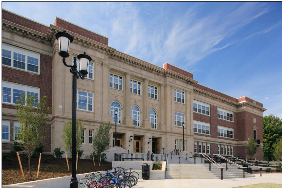
Nathan Bishop Middle School in Providence, RI is one of the first high performance historic renovations in the country. Image courtesy of Ai3.
