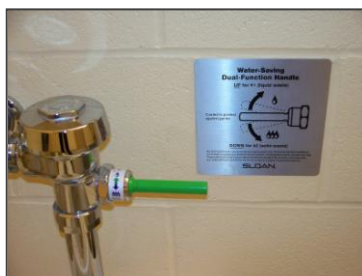
Dual flush toilet at Profile School, NH. Image Courtesy of NEEP.
