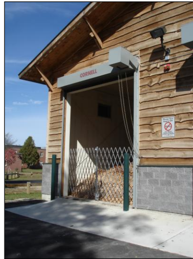
Merrimack Valley HS, NH has a wood chip heating plant that provides heat for the high school and middle school.
