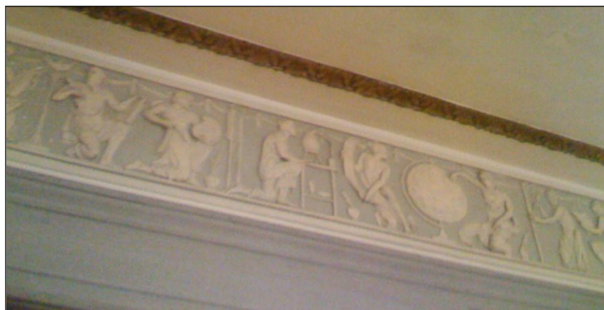
Decorative frieze preserved during the historic renovation of Nathan Bishop Middle School in Providence, RI.
