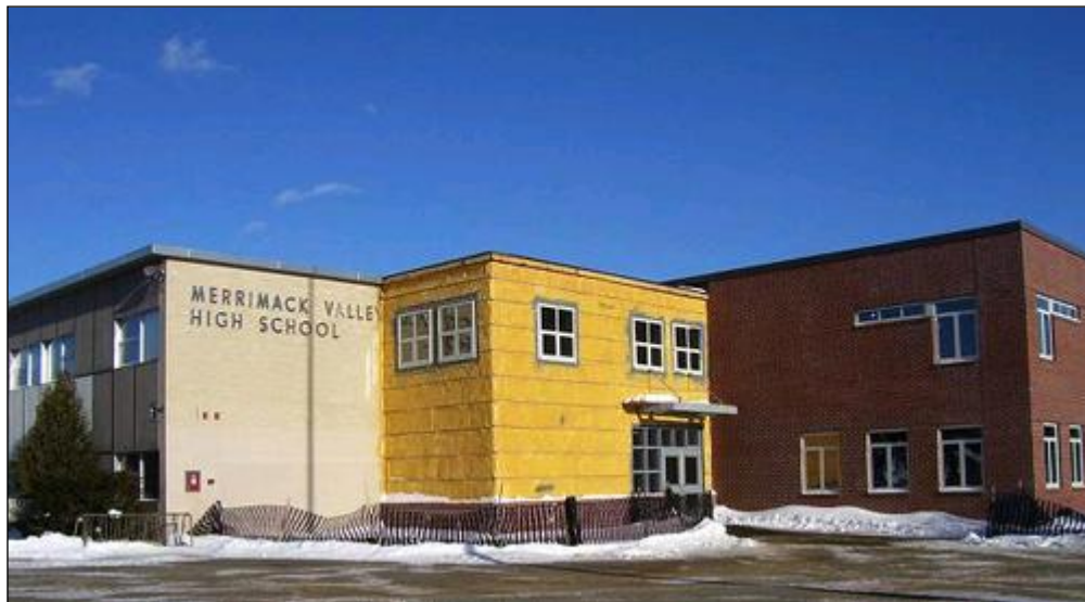
In this picture of Merrimack Valley High School, NH, you can see (l-r) the old building envelope under construction and the new exterior. Image courtesy of Banwell Architects.
