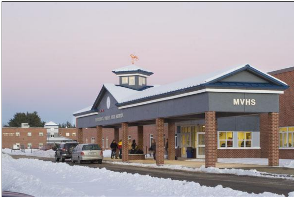
Merrimack Valley High School in Penacook, NH was the first NE-CHPS school building. Image courtesy of Banwell Architects.
