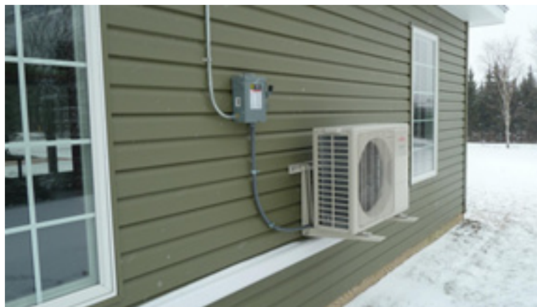
Figure 25. An inverter-driven ASHP in a snowy climate.
