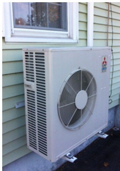
Figure 6. Cold-climate ASHPs operate at low temperatures, so it is important to keep outdoor units elevated and unobstructed from snow and ice.
