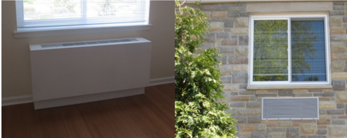
Figure 3. A packaged, terminal heat pump (PTHP) from inside and outside.
