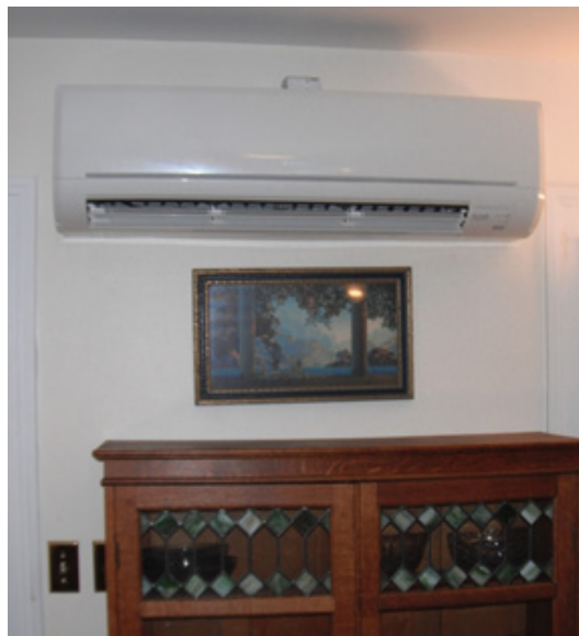
Figure 1. A ductless heat pump fan coil
