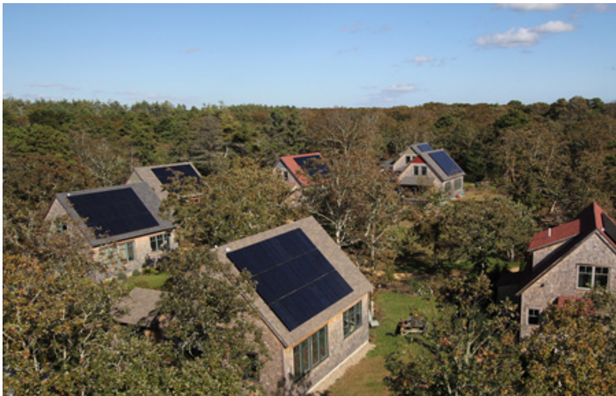
Figure 7. These Eliakim’s Way homes (built by South Mountain Company) are heated primarily by ductless heat pumps. Several homes achieve zero net energy (credit: South Mountain).
