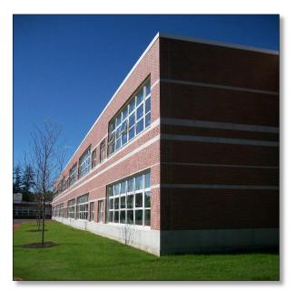
The school addition was designed to optimize natural daylight while avoiding glare. Daylight and occupancy sensors monitor all the spaces in both the new addition and the existing school to adjust the artificial light accordingly.
