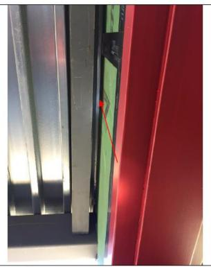
The ZIP sheathing can be spray foamed to the steel plate from the outside to connect the roof AVB to the ZIP sheathing. Kit foam would be best for this small application.
