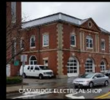
CAMBRIDGE ELECTRICAL SHOP
