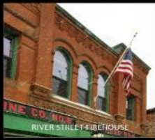
RIVER STREET FIREHOUSE
