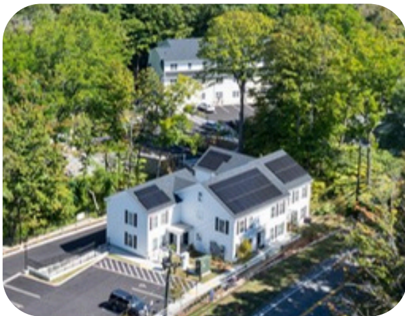
Front building (Building 20), a 6-unit ENERGY STAR® certified building, and rear building (Building 22), a 28-unit building certified under Phius Core 2021.
