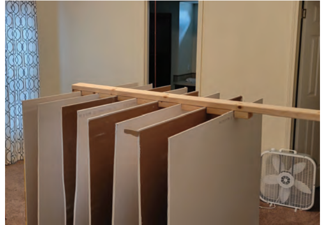
Figure 2-11. Drywall sheets installed in “bedroom 1”
