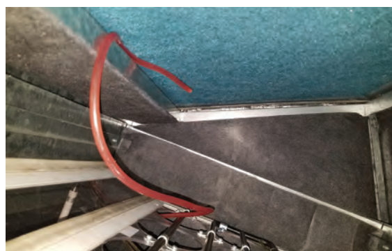
Figure 2-57. Probe location for inlet, system A
