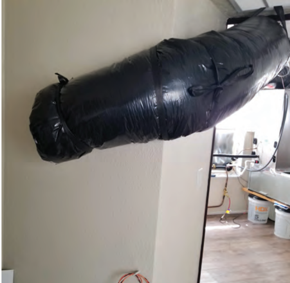
Figure 2-12. Ducted HP ductwork ends in utility room facing native furnace return
