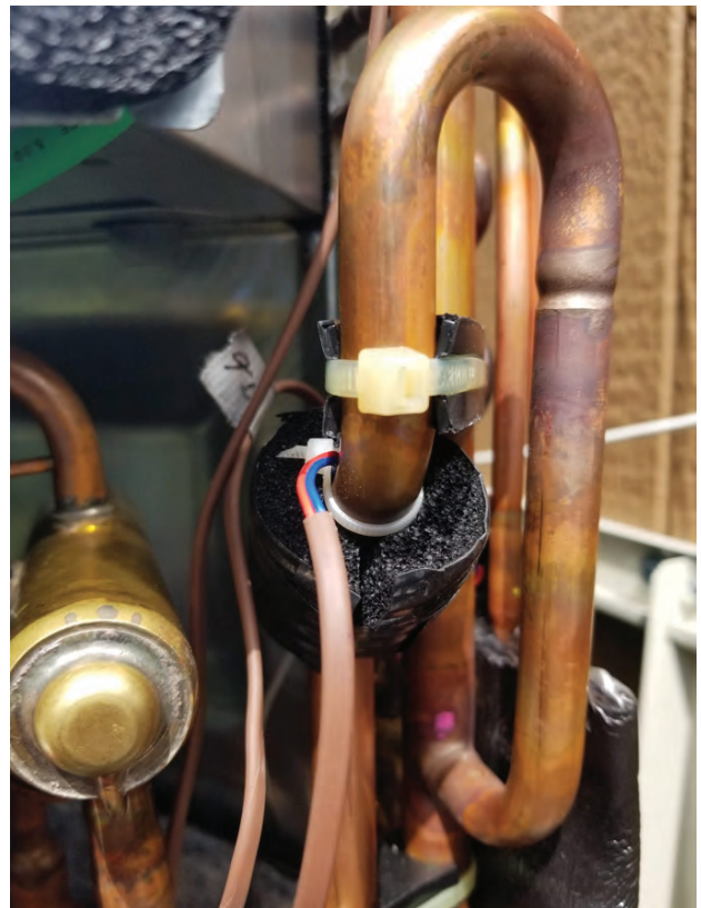
Figure 2-51. Ductless HP thermocouple, true suction
