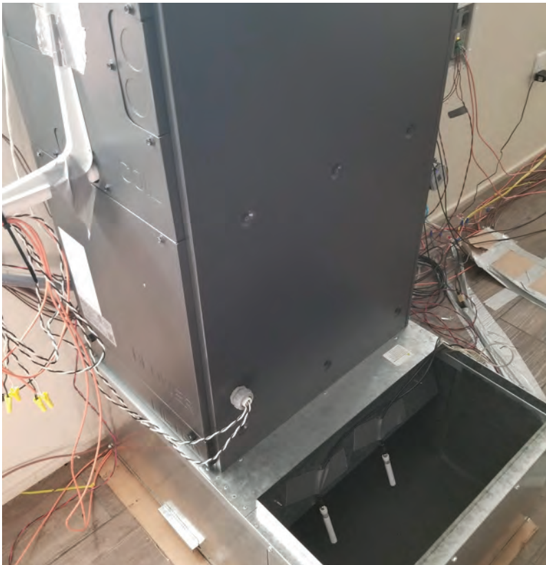
Figure 2-43. Ducted HP inlet air temperature sensor location
