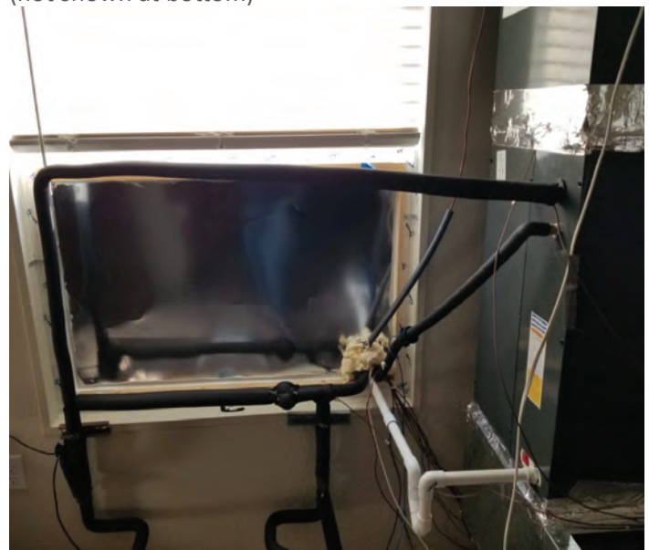
Figure 2-24. System B indoor let set and mass flow sensor (not shown at bottom)
