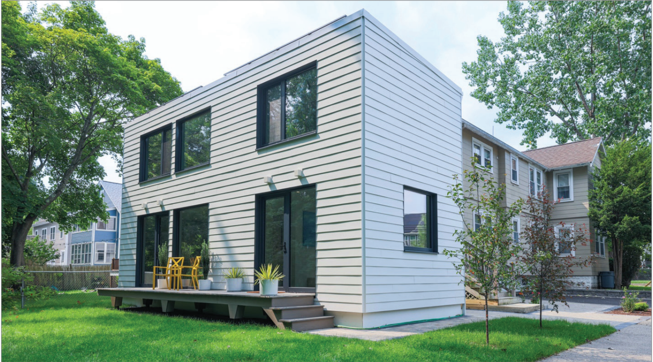
Figure 4. Completed ADU installed at the site.
