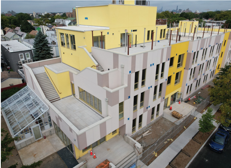
Figure 6. Bethany Senior Terraces under construction.
