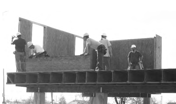
Figure 7: SIPs on-site installation, photo by C. Wu, NEEP
