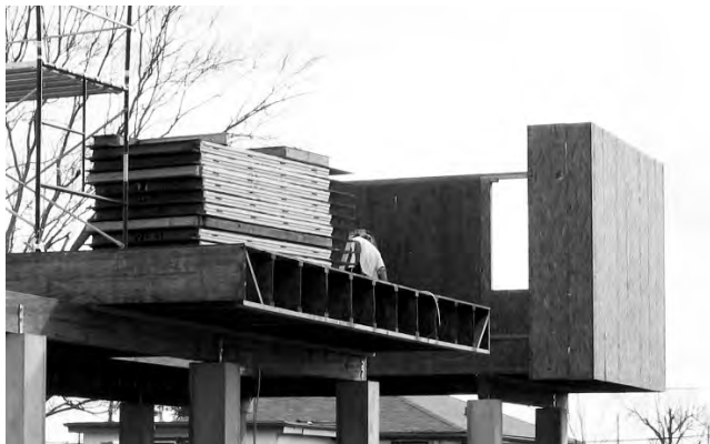
Figure 6: SIPs on-site installation, photo by C. Wu, NEEP
