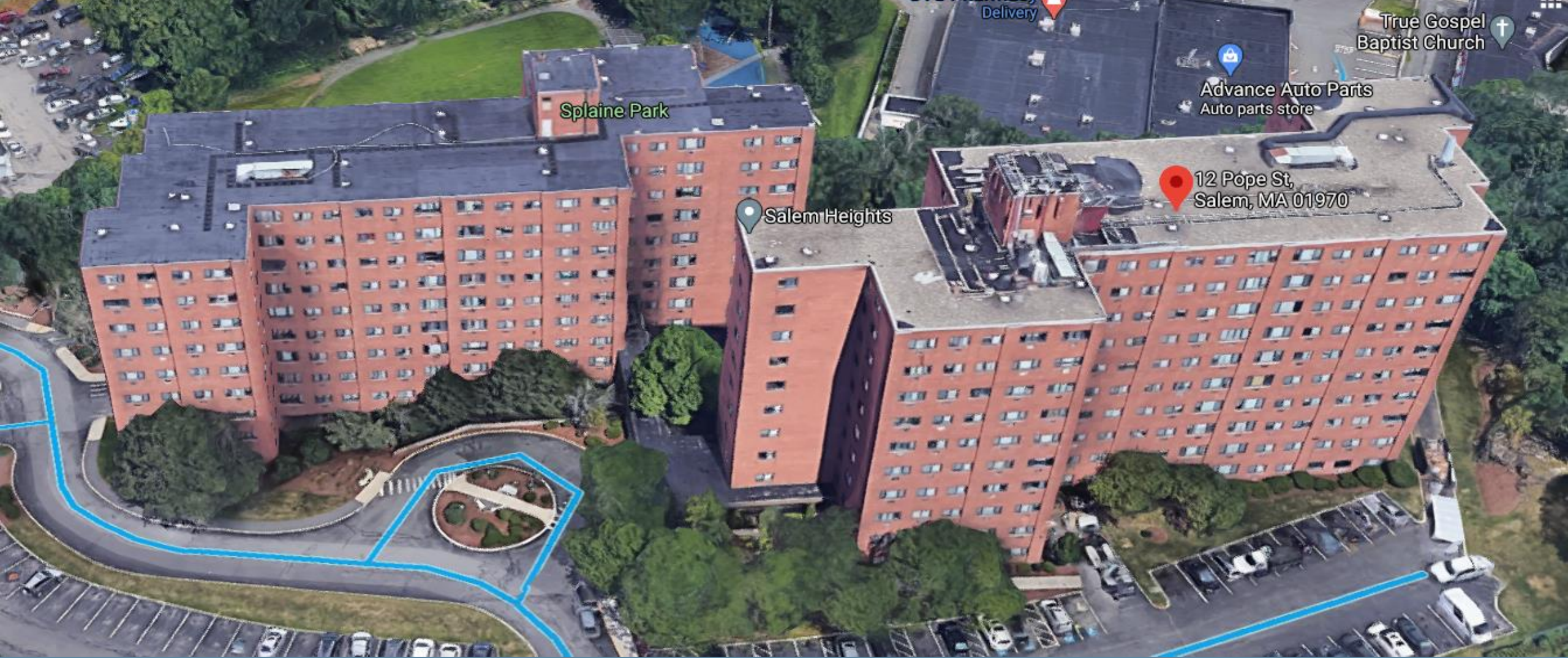
Salem Heights, 281 Units Family, Salem, MA Built: 1974
