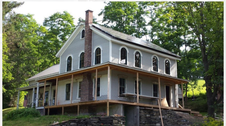
Figure 2: Barden Seidman Residence near Complete Renovation, 2017
