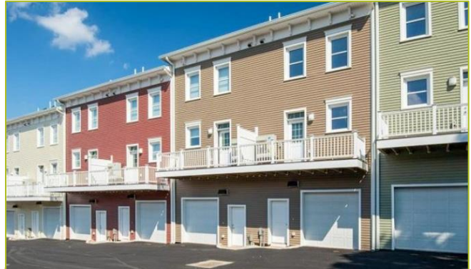
Crown Street by Hanes Construction is a three-bedroom, three bathroom (1000 ft 2 ) certified ZERH located in Connecticut. The building is part of the municipality’s affordable housing program. The annual energy savings of this home are estimated at $2,950. The HERS index for this home is 31 (without PV).
