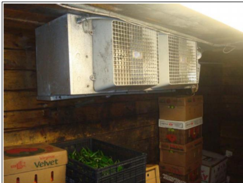
Figure 7. Example of Two Evaporator Fans in a Walk-in Cooler
