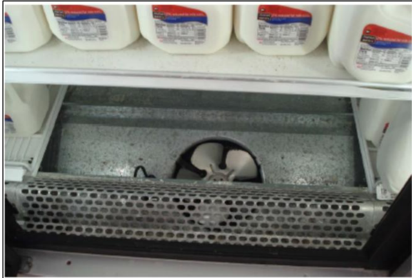
Figure 8. Example of Evaporator Fan in a Reach-in Cooler
