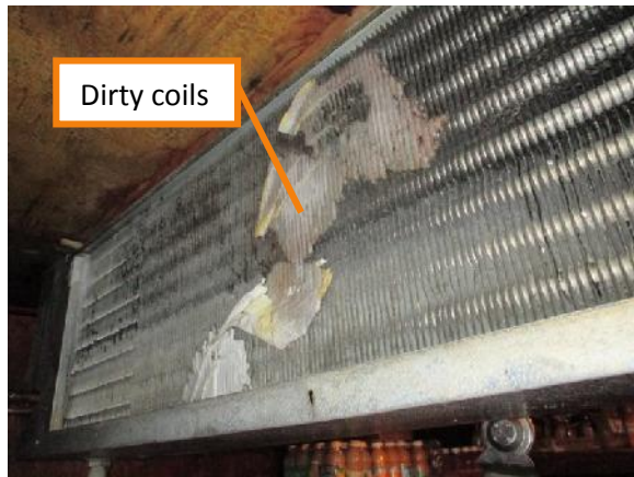
Figure 56. Examples of Poor Evaporator Coil Conditions
