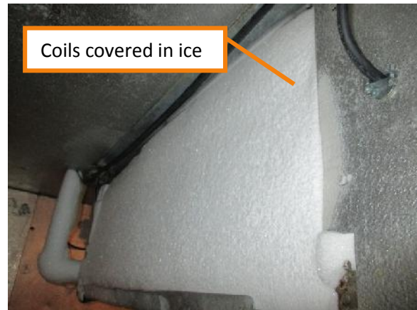
Figure 56. Examples of Poor Evaporator Coil Conditions
