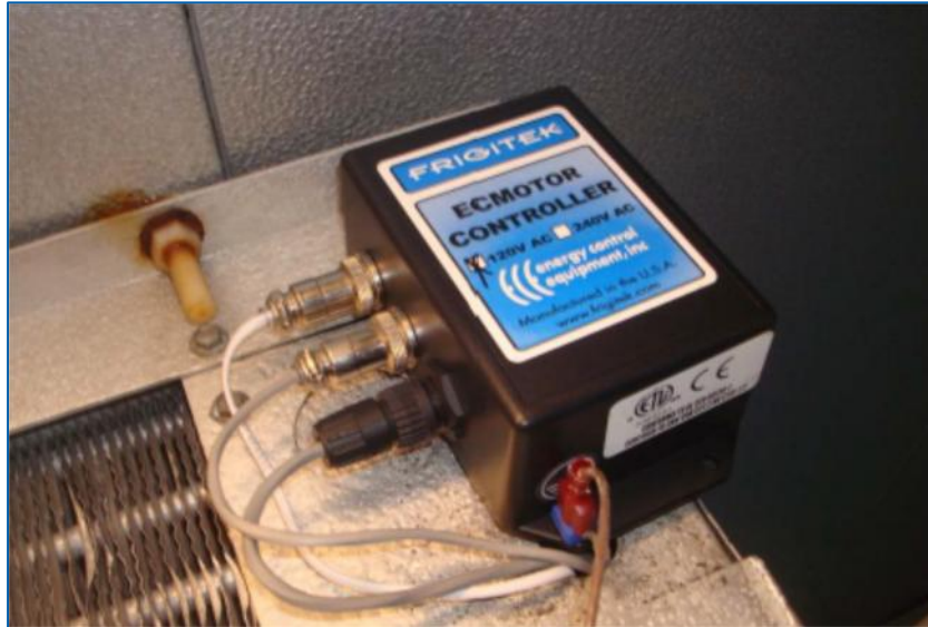
Figure 11. Example of EF Controller for ECM
