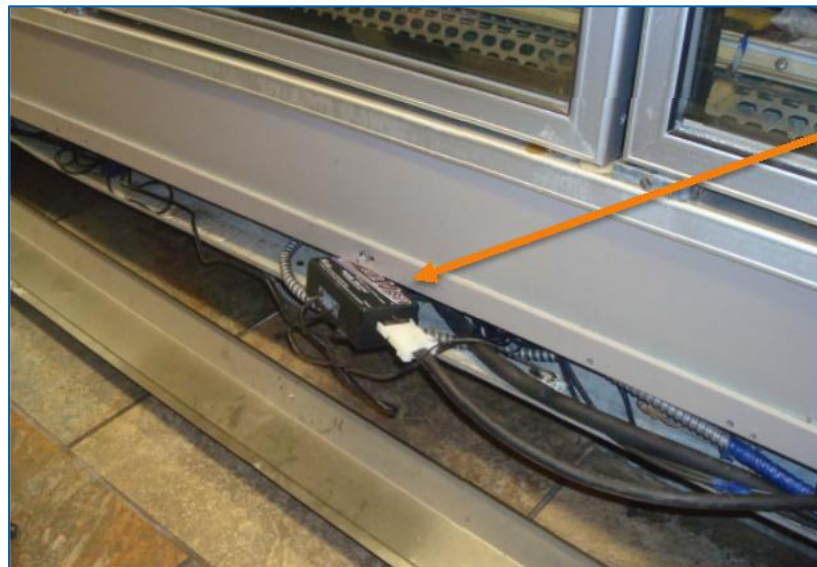
Figure 14. Example of ASDH Control Installed on Reach-in Case
