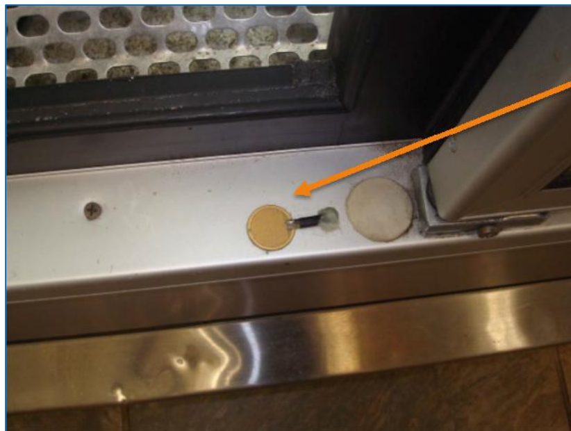
Figure 15. Example of Moisture Sensor for ASDH Control
