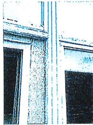
SINGLE GLAZED WINDOWS AND RUSTING STEEL FRAMES
