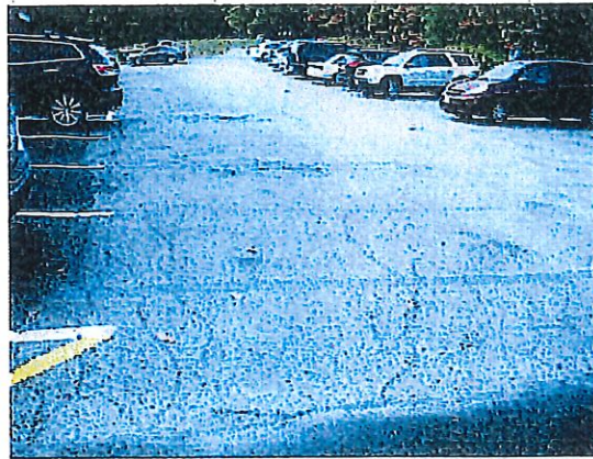
FATIGUE CRACKING AND HEAVING/SETTLEMENT IN NORTH PARKING LOT
