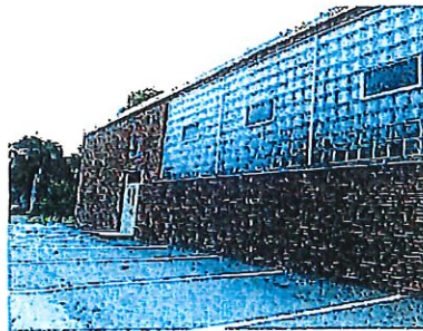
BRICK AND GLASS BLOCK REPOINTING REQUIRED
