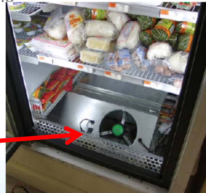
ECM Motor, before blade is installed.
