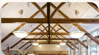
Salvaged wood truss
