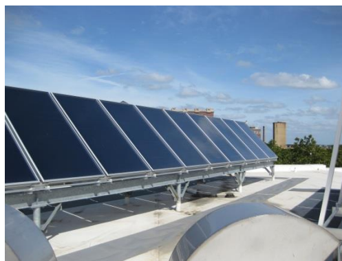
Solar panels at Providence Career and Technical Academy in Providence, RI
