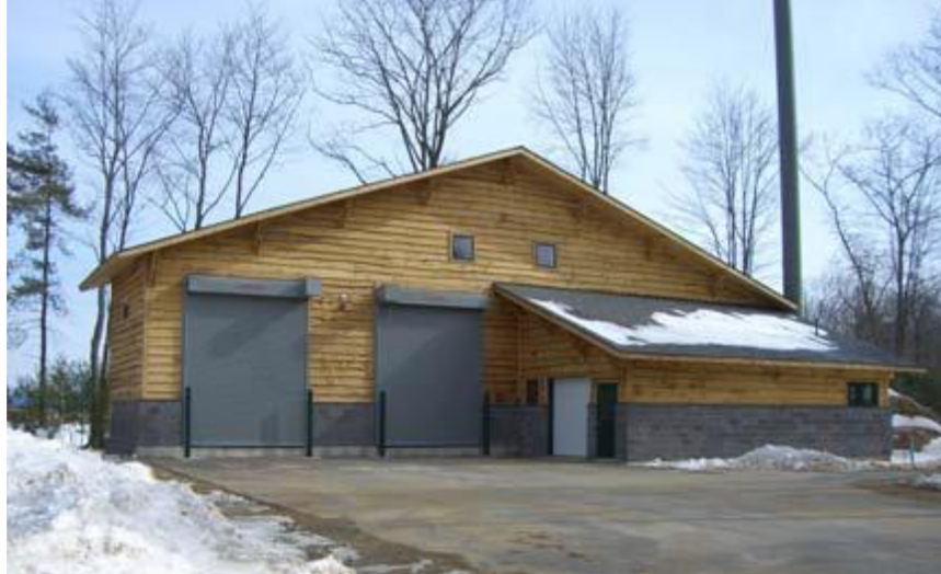
Figure: Exterior view of Merrimack Valley Regional High School (Pennacook, NH) Wood Chip Heating Plant. The smaller building near the entrance of the plant serves as the observation learning space for students and visitors.
