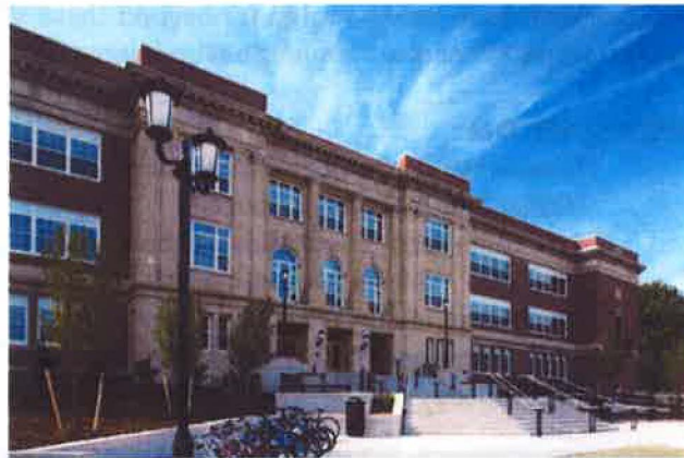
Nathan Bishop Middle School, Providence, RI is the first NECHPS historic renovation.
