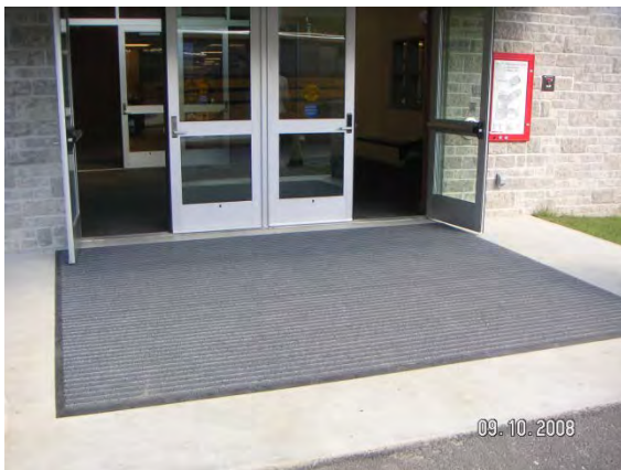
Walk off system at New Hampshire school
